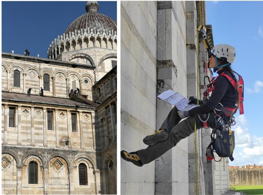
Fig. 1-2 The conservator is mapping critical areas on the architectural survey while suspended by ropes.
