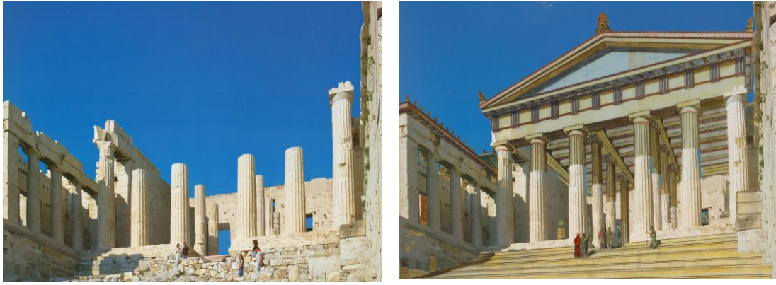
Fig. 1. Propylaea, Acropolis: elaboration of the monument's architectural survey and its graphic representation (G. Antoniou, 2008, Ancient Greece. The Monuments then and now , p. 12, Propylaea depicted before restoration works).
