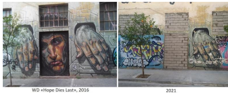
Fig. 6. WD's mural adapted to the building concerning its historical and social value and intervention by city authorities.
