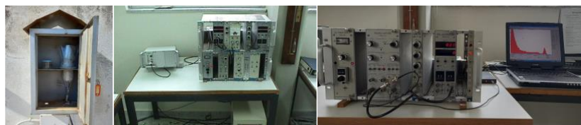
Figure 1. Left: The 2"x2" NaI detector mounted on the building wall. Center: The original setup electronic configuration. Right: The signal processing and storage units currently in use.
